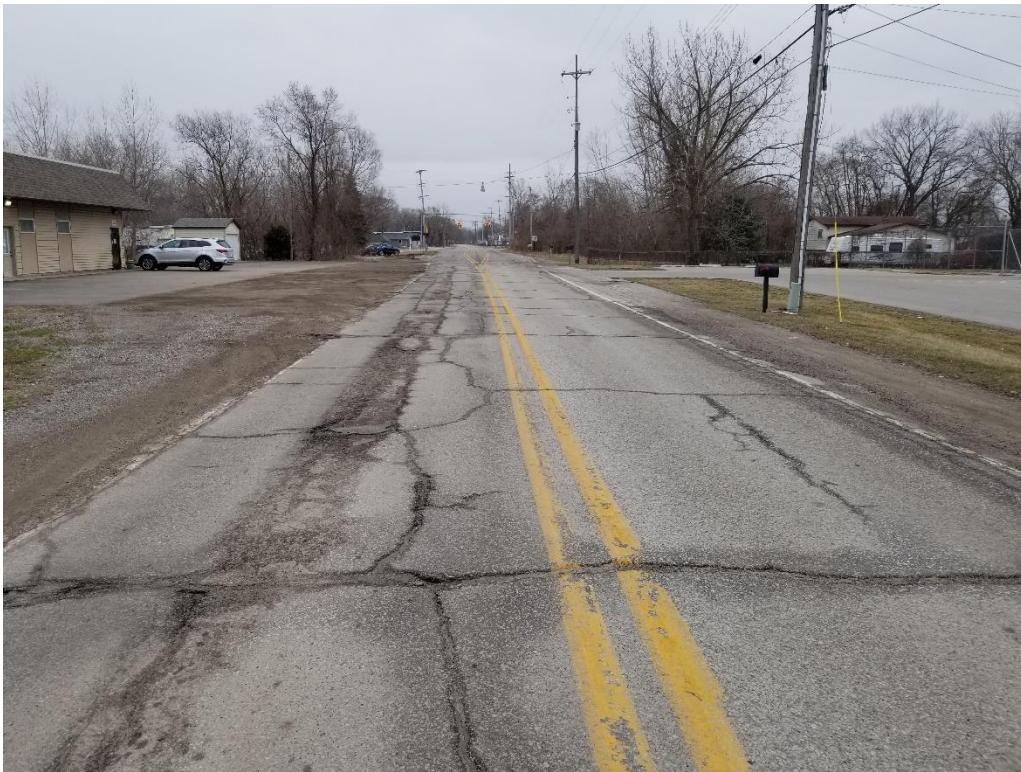
Before Construction (Looking East from Wheeler Rd)
